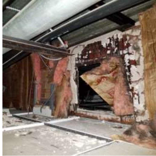
Plaster at east overhang area, not asbestos
