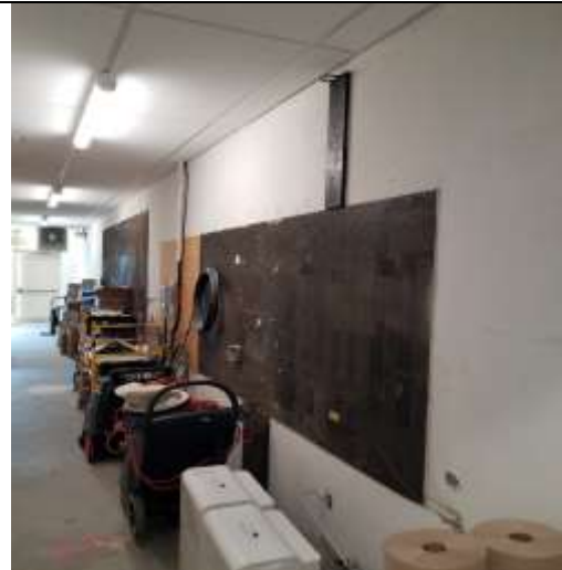
Outer south wall, not removed, asbestos JC
