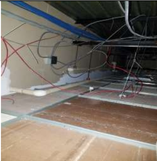
New gypsum board in plenum
