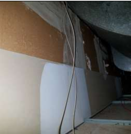
Double layer gypsum/JC in S/E kick out hall
