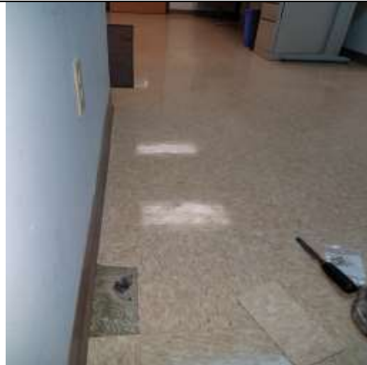
S/E vacant section new floor tile
