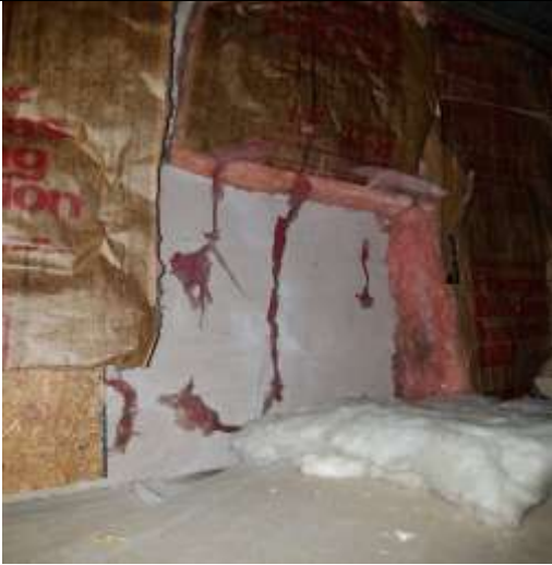
Red insulation sealer glue, not asbestos
