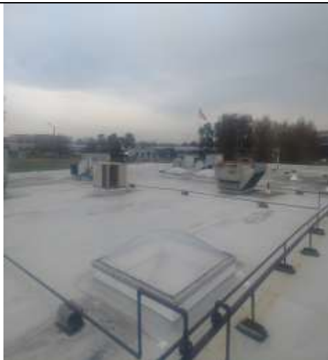
View of roof
