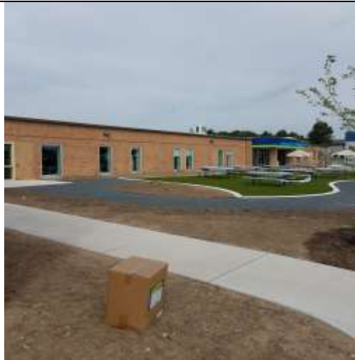
General exterior front view
