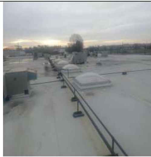
View of roof
