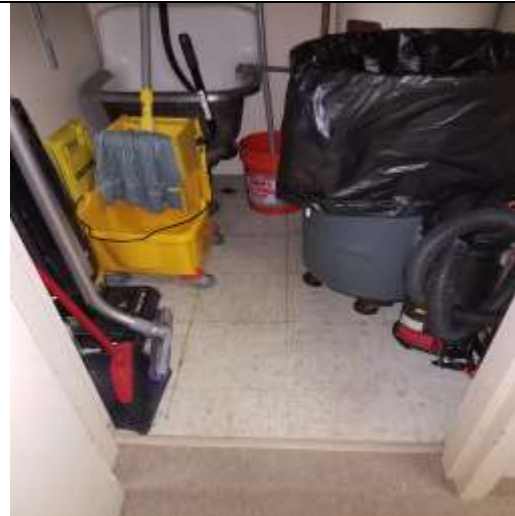
Janitor closet 2071, asbestos floor tile/mastic
