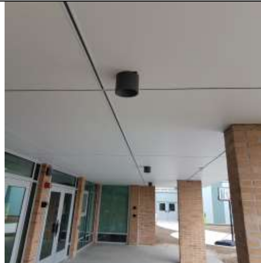
Main entrance gypsum overhang
