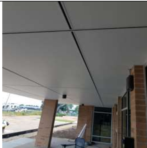
West entrance overhang is gypsum panels
